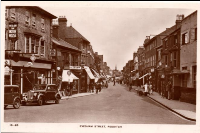
Above: Evesham Street looking north from the junction of George Street (right). All of these buildings were demolished in the 1970's to make way for the southern part of the Kingfisher Centre. The garage on the left is approximately where Primark is situated.
